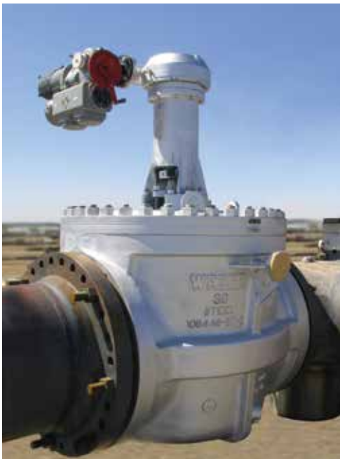
WEDGEPLUG™ installation at Suncor Millennium 2 Coker project, Fort McMurray, Alberta Canada. Electrically actuated 30" full port WEDGEPLUG™, overhead vapor line isolation service.
